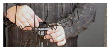
The last step is to add the pendant lamp wiring. Insert the lamp holder from the bottom and screw on the retaining ring. Add a bulb and give it a test!
